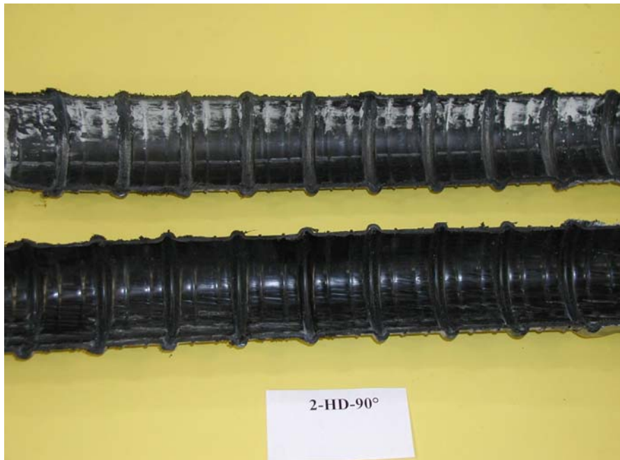
Figure 4-20 Damage in specimen 2-HD-90°
