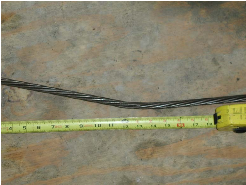
Figure 4-8 Sharp bend on strand
