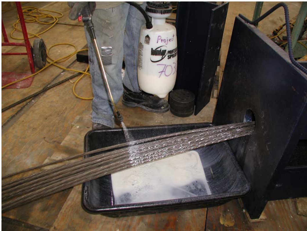
Figure 3-19 Oiling of tendon
