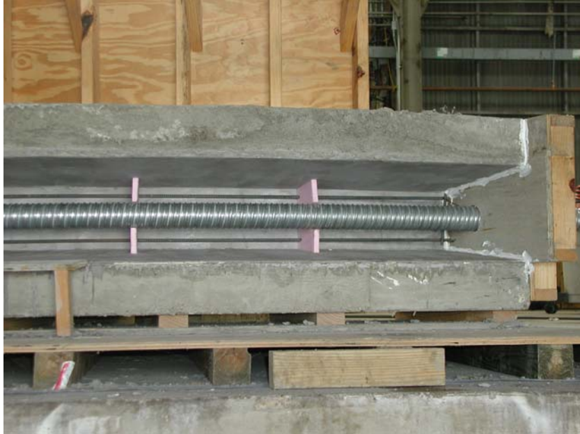
Figure 3-12 Installation of galvanized steel duct
