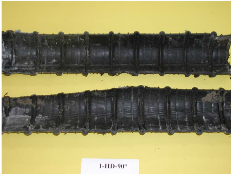
Figure 4-19 Damage in specimen 1-HD-90°
