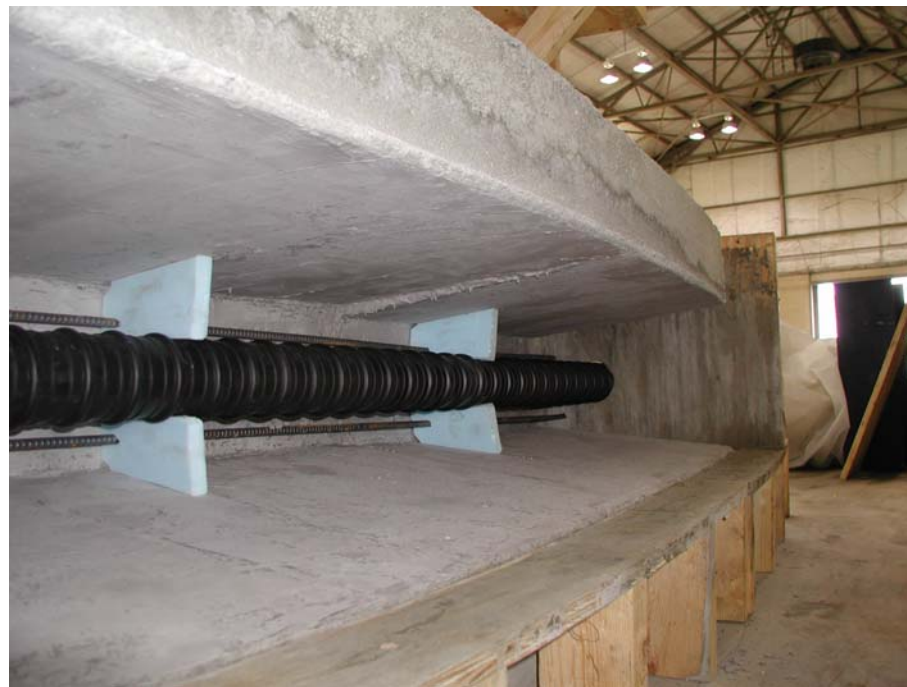
Figure 3-11 Installation of HDPE duct
